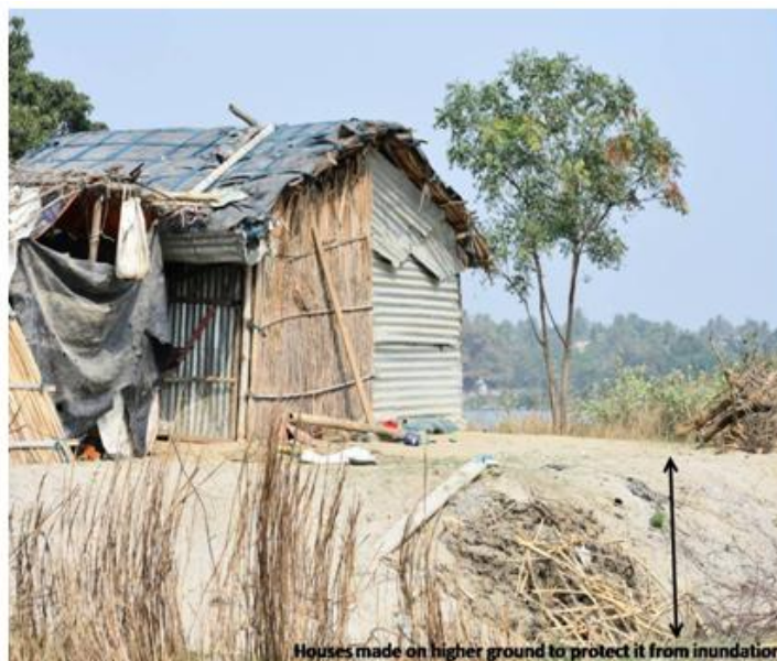
Plate-6: Houses built on elevated surface to protect it from water inundation
